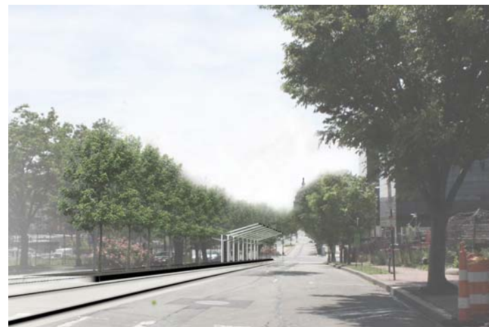
View Across Stop & Alignment
